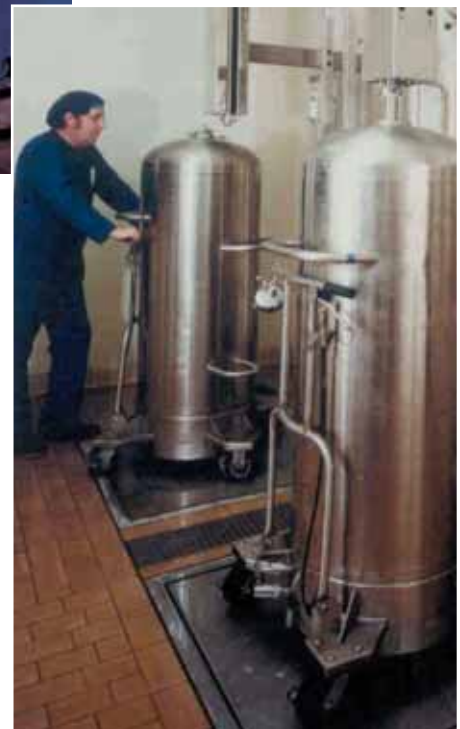
Weigh filling: Coca-Cola syrup is filled by two Masterfil machines at Golden West Foods
