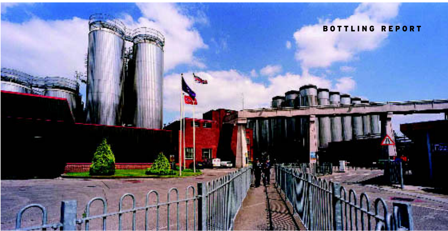
Coors' Burton-on-Trent brewery: The Merlin project aims to minimise whole life costs for the revised packing lines rather than just the initial expenditure
